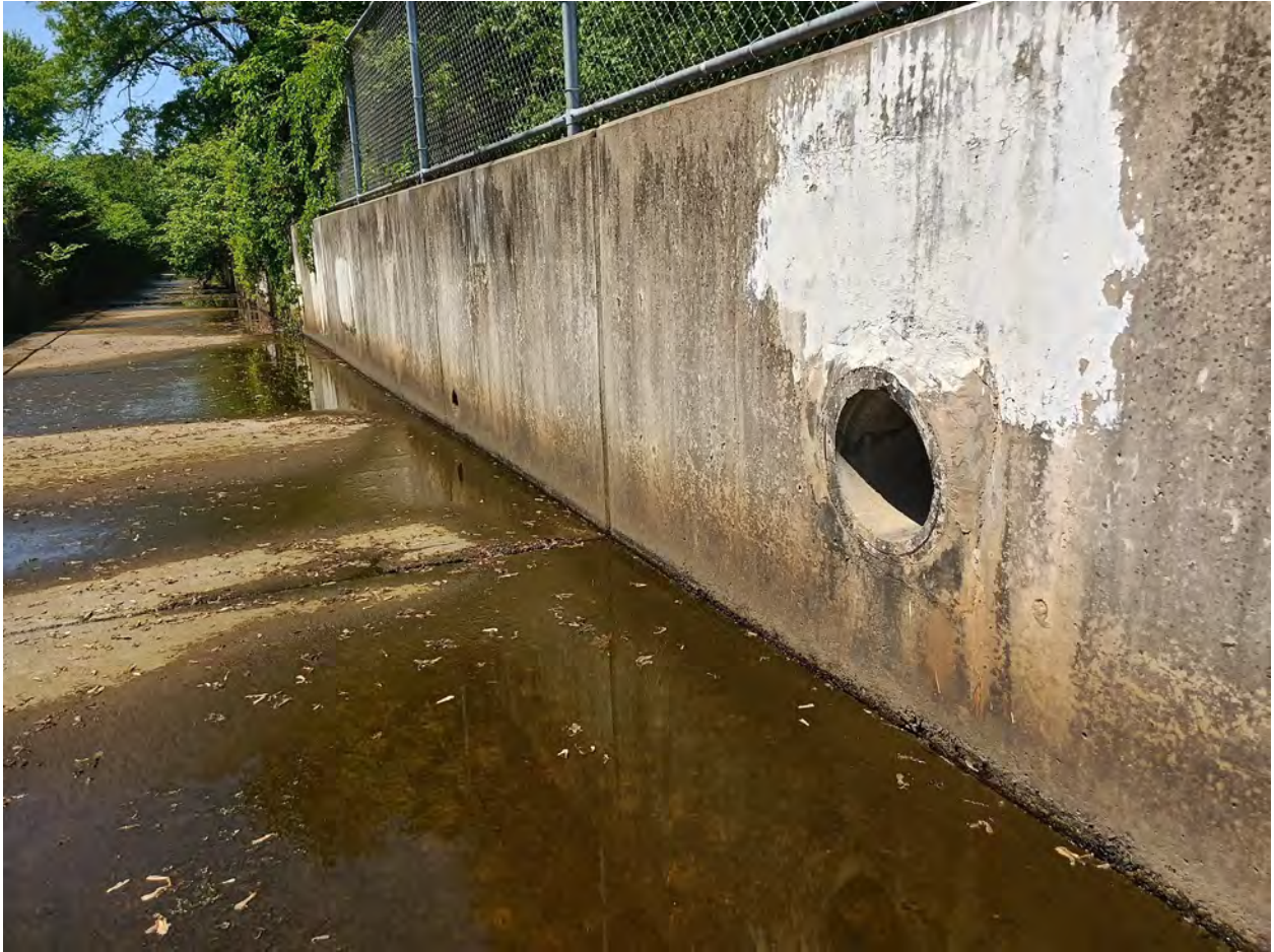
Outfall ID #E0315
