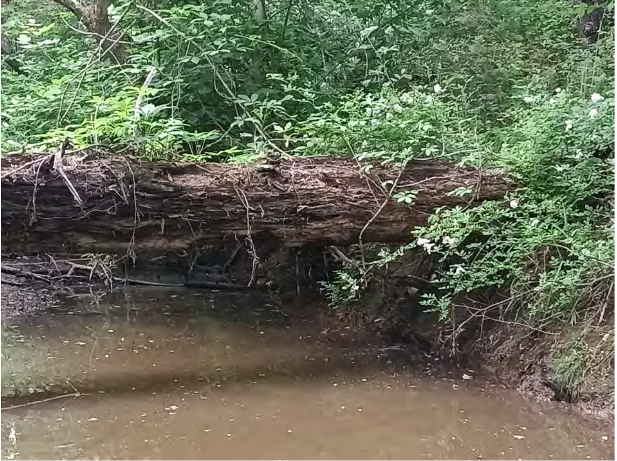
Outfall ID #89 - no outfall pipe located
