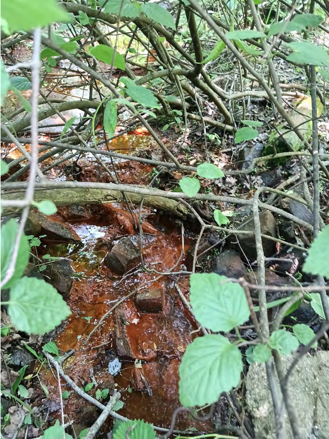
Outfall ID #44 - no outfall pipe located
