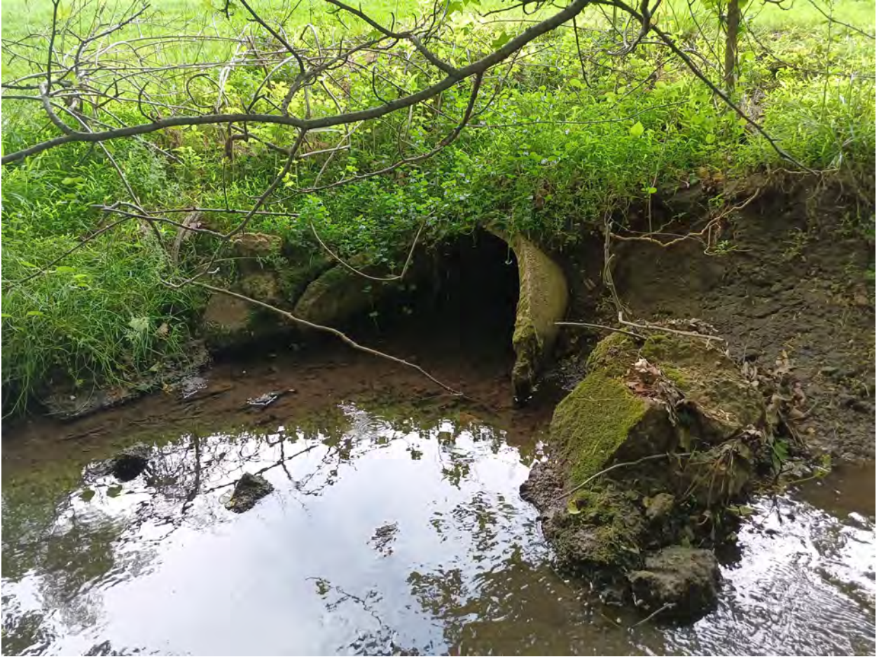
Outfall ID #B0326
