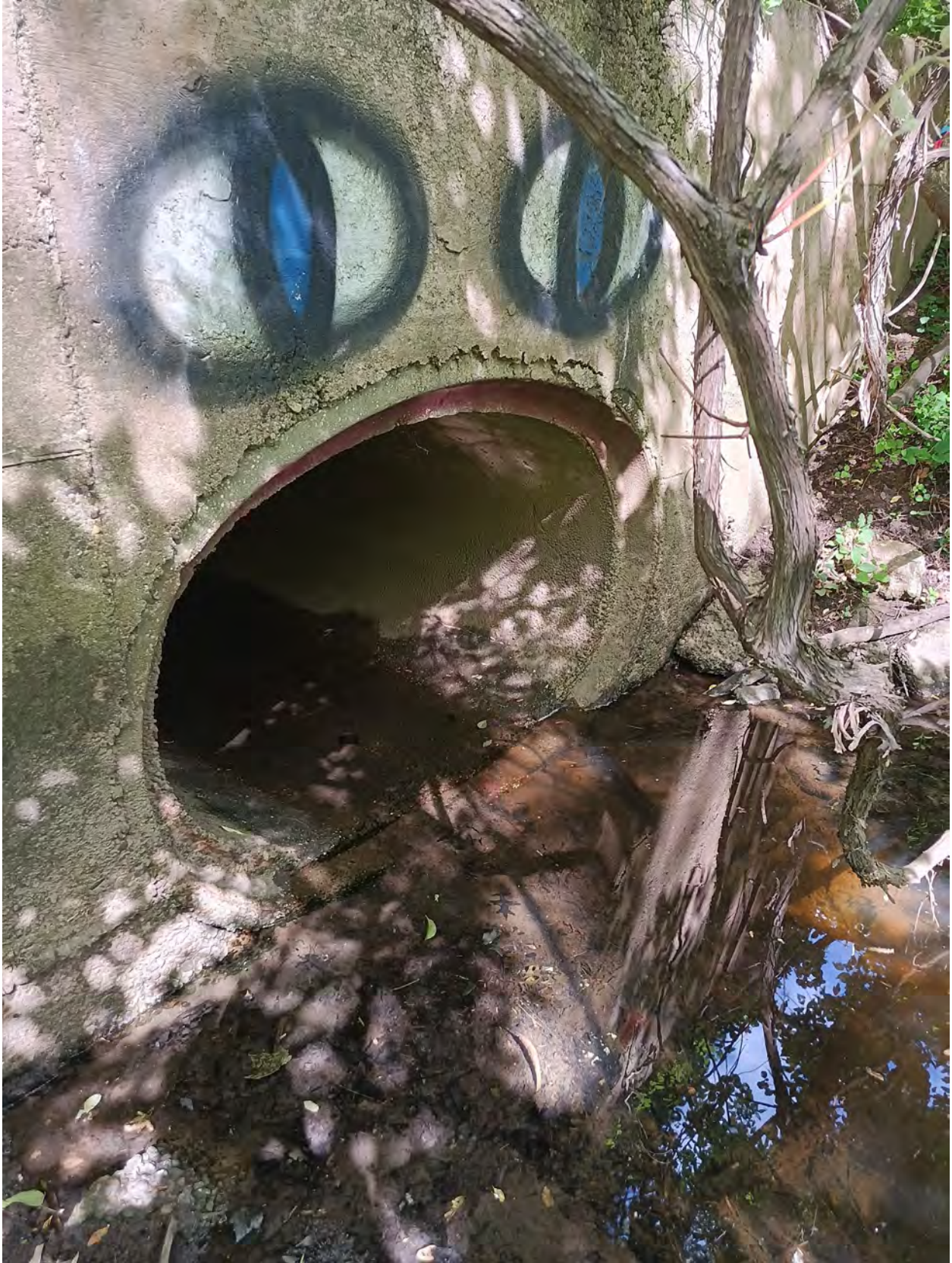
Outfall ID #B0329
