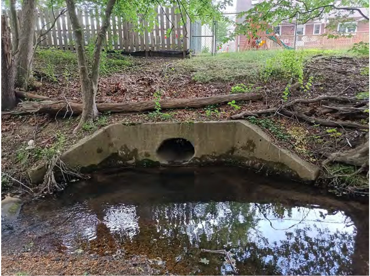
Outfall ID #B0307
