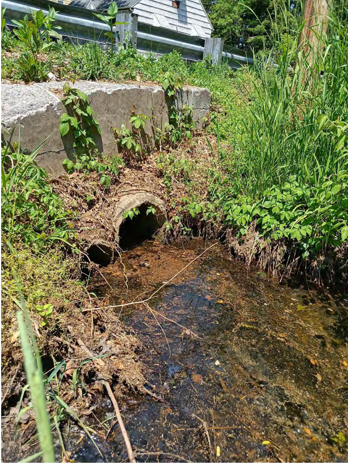
Outfall ID #B0303 & #BO304
