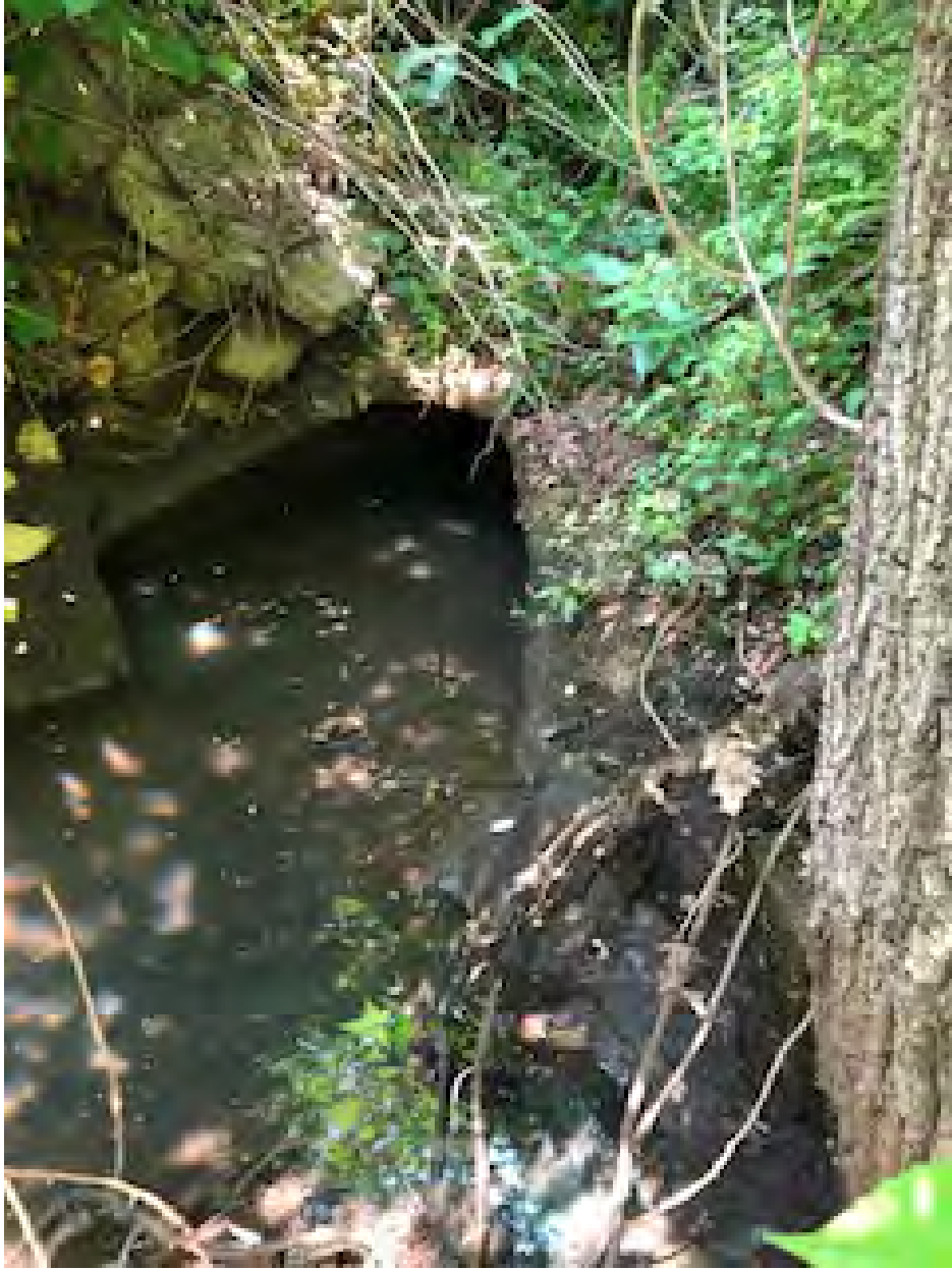
Outfall ID #G505
