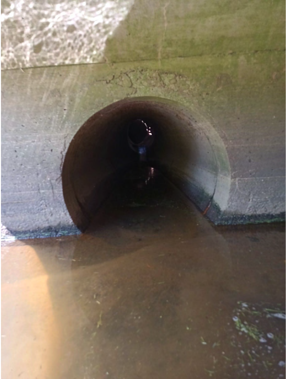
Outfall ID #B0401
