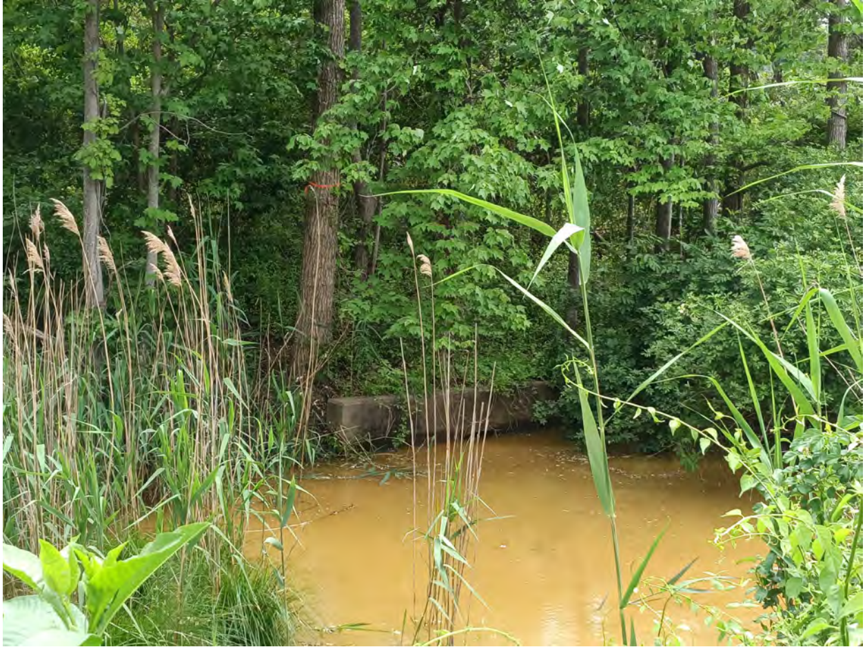
Outfall ID #D0211 (only headwall visible)
