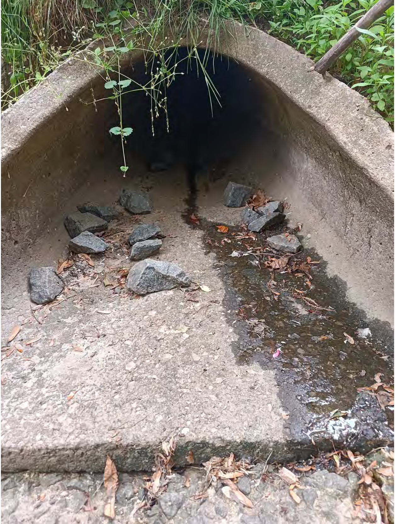
Outfall ID #B0306
