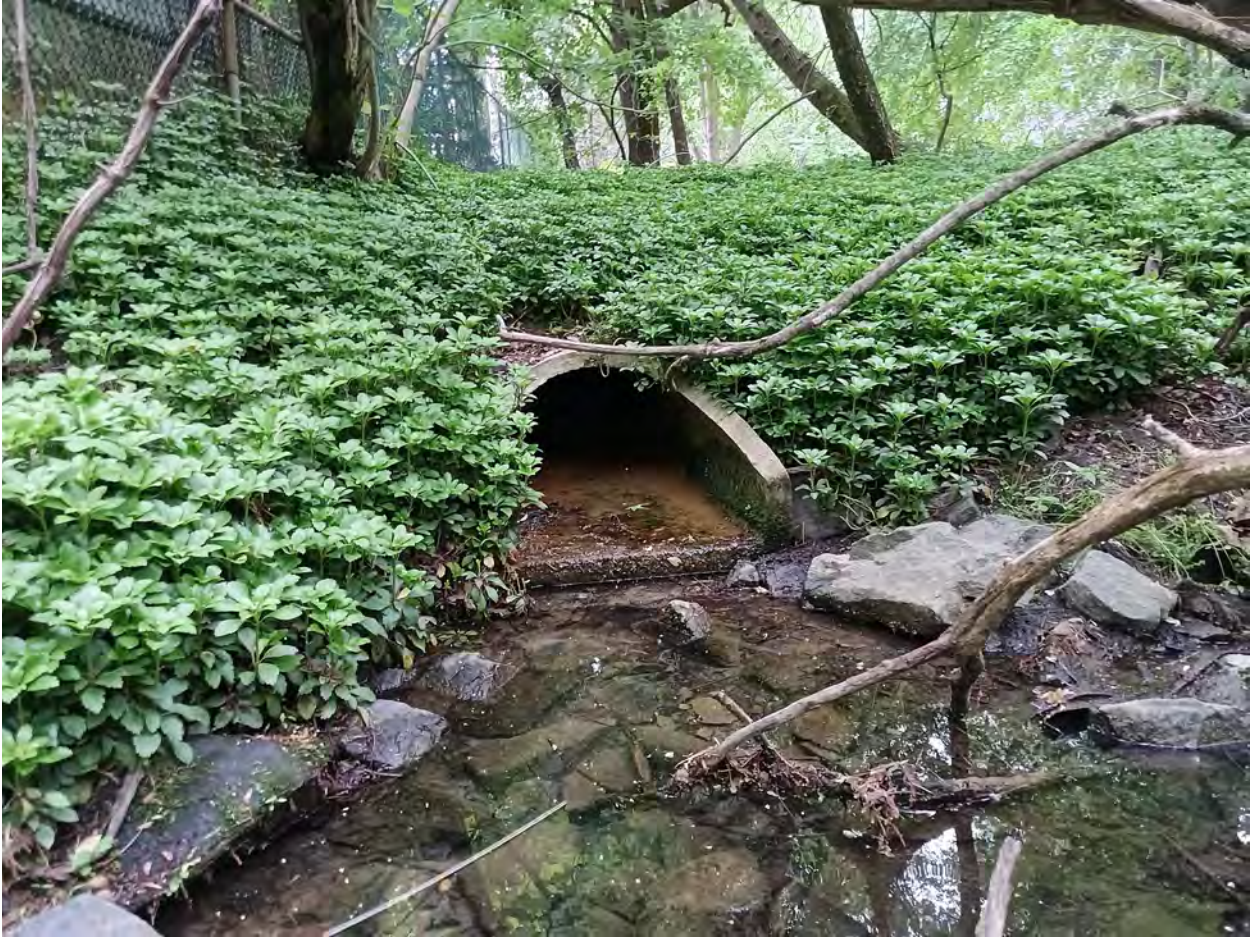
Outfall ID #B0311
